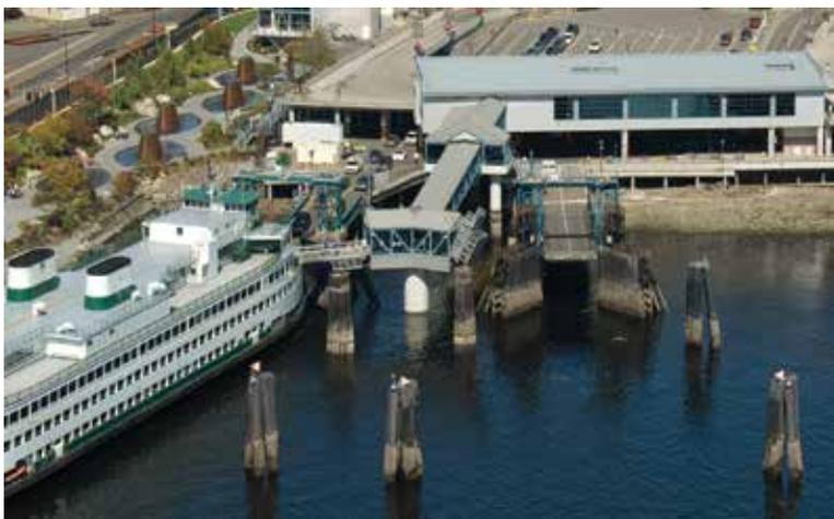
This photo shows WSF typical dolphins, wingwalls, transfer span, and passenger overhead.
